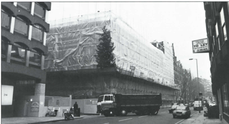
Ready for demolition
