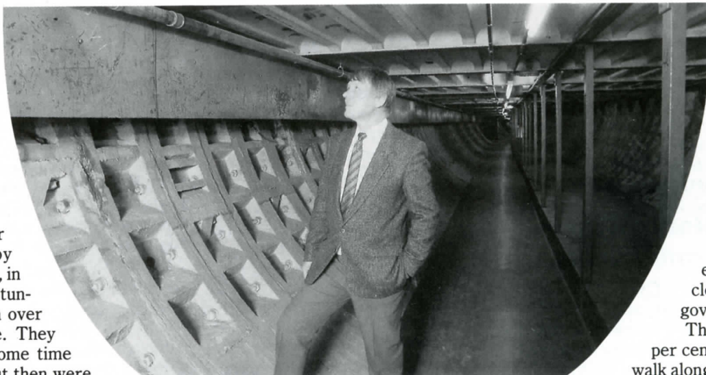
Upstairs, downstairs: the tapes are in the upper level but the lower is a reminder of its previous use.
